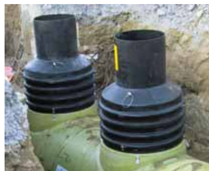
A special-shaped gasket guarantees the maintenance shaft is tight.
